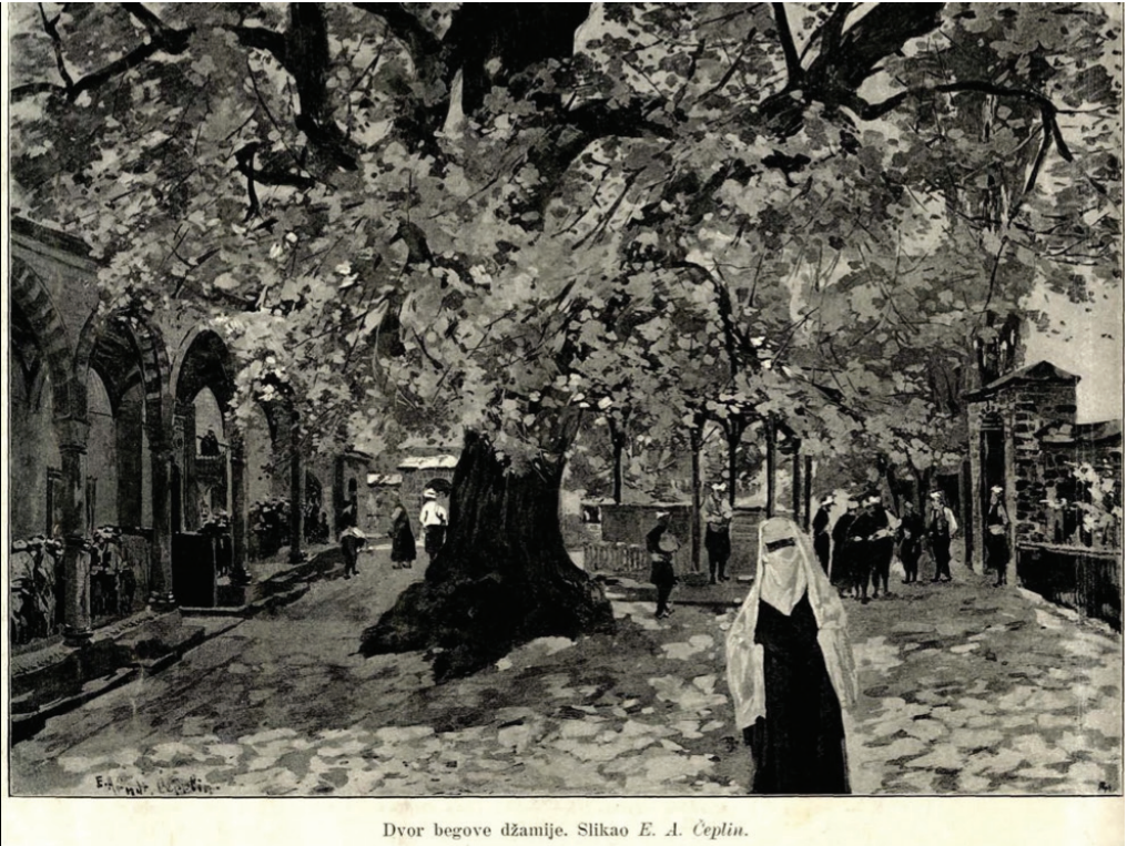
FIGURE 3. E.A. Tschepelin, 'Harem or Courtyard of the Gazi Husrev-bey mosque', Nada 1: 8 (1 January 1895). ©Gazi Husrev-bey Library, Sarajevo
